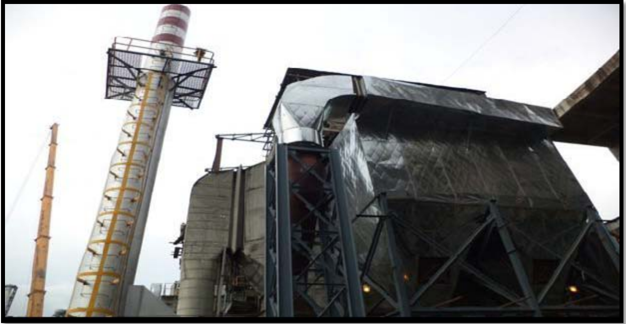
Cement Mill-2 Bag filter
