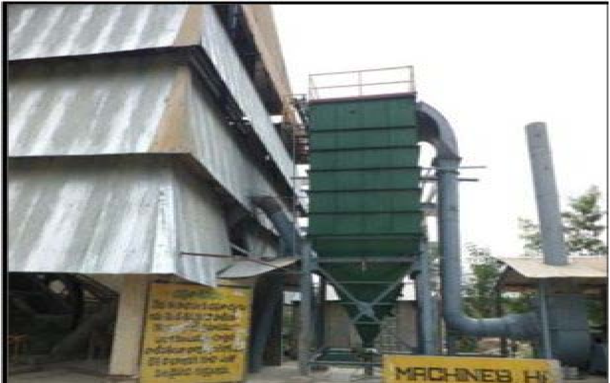
Bag Filter Installed on Crusher
