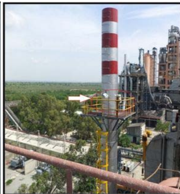
CEMS Analyzer on the Cement Mill-2 Stack
