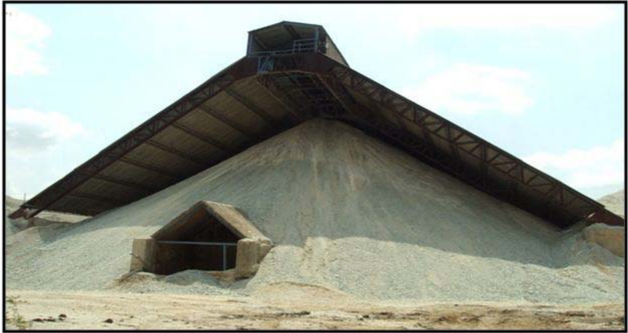
Crushed lime stone yard
