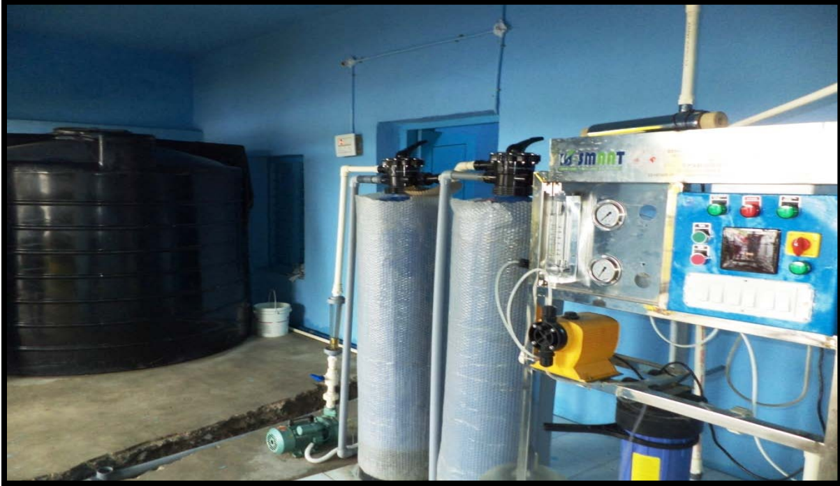
RO Water Plant Provided in Srinagar village
