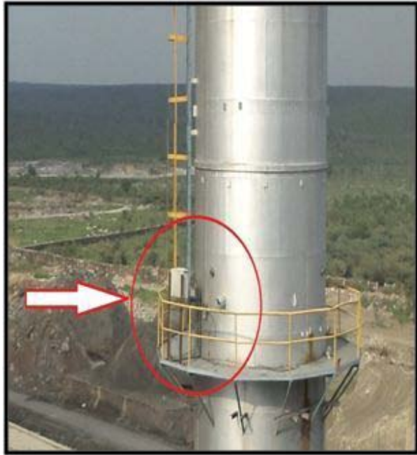
Cooler ESP Stack
