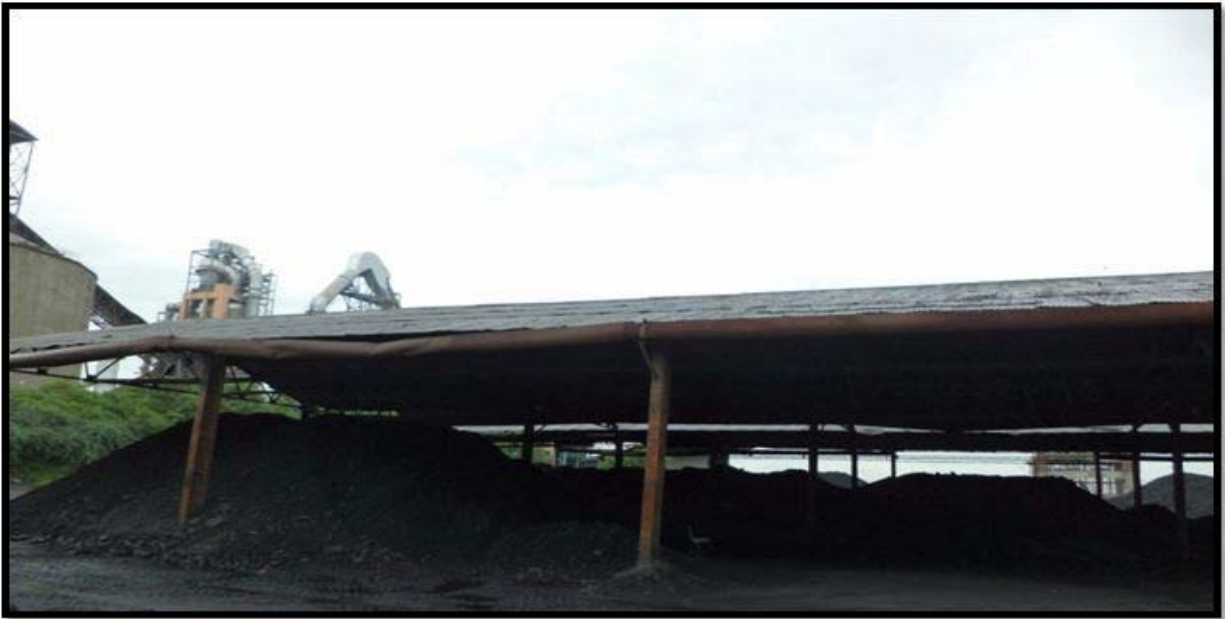
Covered Coal yard
