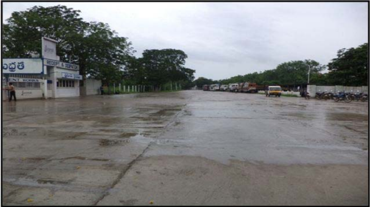
Concreted roads provided and maintained
