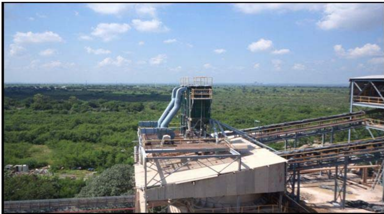
Tree Plantation inside the factory premises
