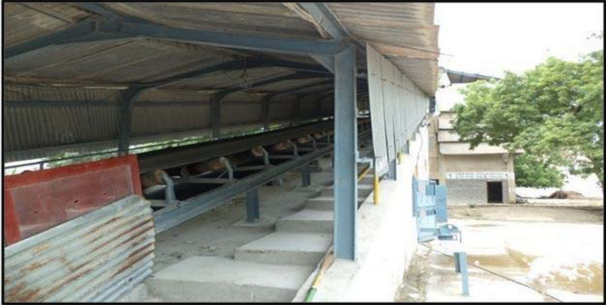
Covered belt conveyors
